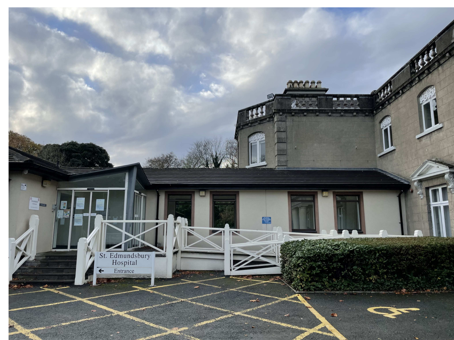
Link corridor between St Edmundsbury Historic House and the 52 bed In-Patient Facility
